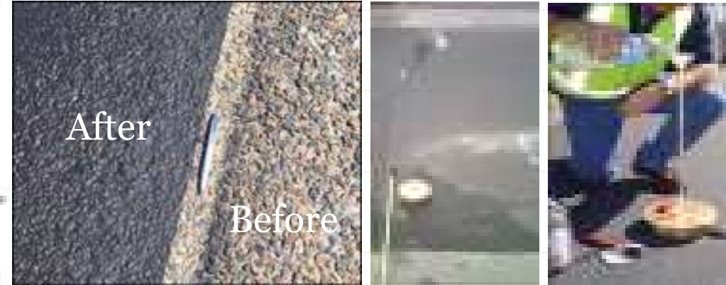
PME applied to stripping seal Permeability testing RTA T168
